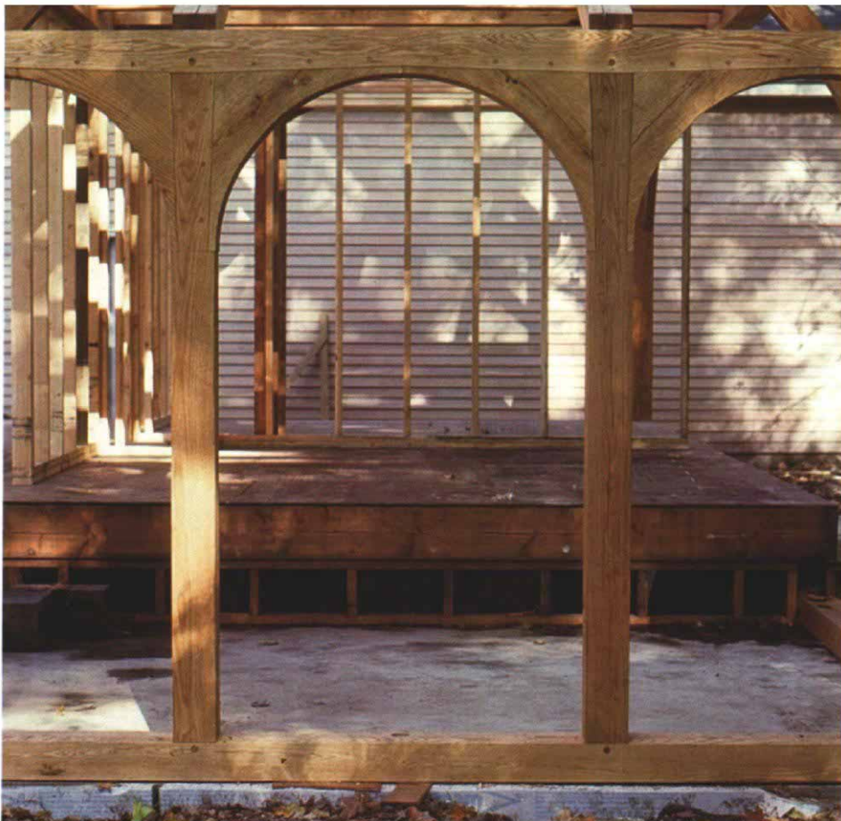
Each arch in this sunroom is made up of two quadrants sawn from wide stock (drawing below). The 5x5 plate waves slightly along its lower edge as it reflects the slope of the arch quadrants. The plate is mortised along its entire length. Photo by Karen Bussolini.
